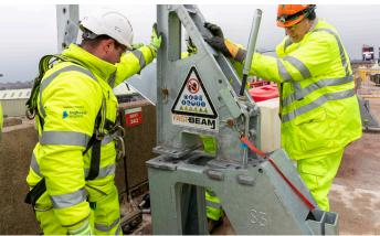
We offer in-house access solutions for all types of structures, including our Fast Beam and V-Deck technologies which provide innovative means of quayside or underdeck access for repair/inspection of marine assets such as jetties, quay walls and lock gates. These technologies eliminate the need for traditionally complex and costly scaffolding.
