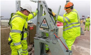
We offer in-house access solutions for all types of structures, including our Fast Beam and V-Deck technologies which provide innovative means of quayside or underdeck access for repair/inspection of marine assets such as jetties, quay walls and lock gates. These technologies eliminate the need for traditionally complex and costly scaffolding.
